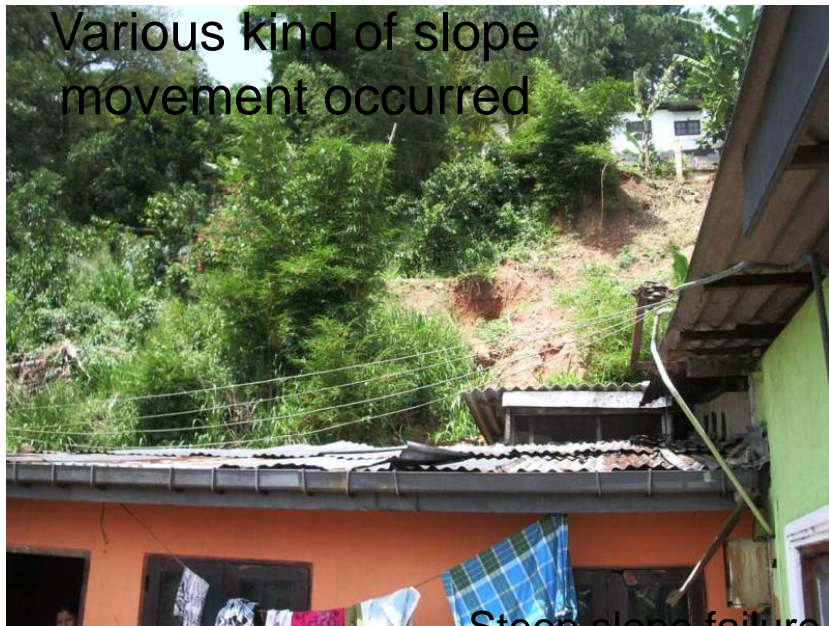
Steep slope failure
